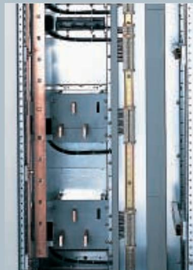
*Plug-on bus system with safe-to-touch protection*
